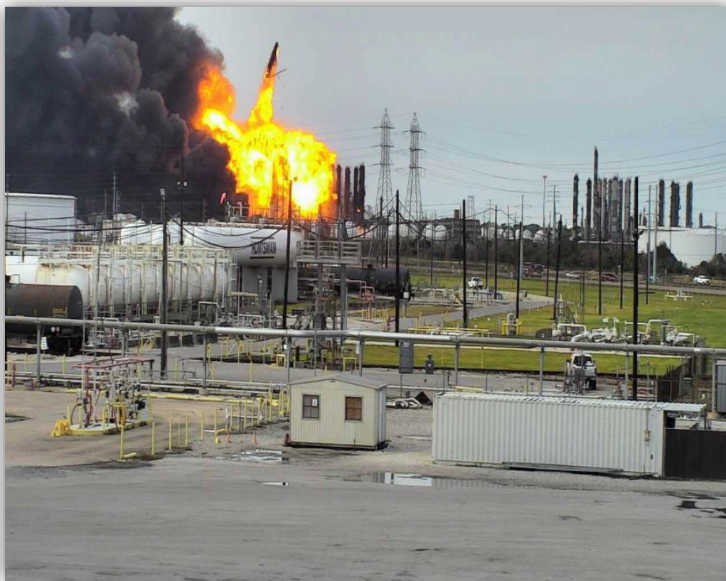
Figure 6: Explosions of PNO facility in Port Neches, Texas in 2019 [6]
