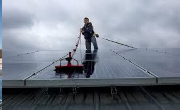
Figure 3: Cleaning using vacuum suction
